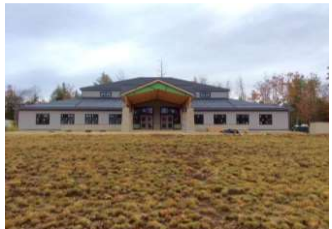
November 2016: The interior rooms are taking shape as electrical, plumbing and drywall contractors apply their handiwork.
